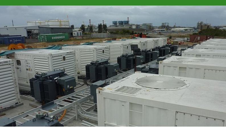
ESE project managed, installed, commissioned and maintained a 30MW power installation in an African region growing rapidly to support the local grid supply. From initial concept, through the design stage we carried out a full site survey working with the client to project manage the set up from design and delivery to site, through to full installation.
